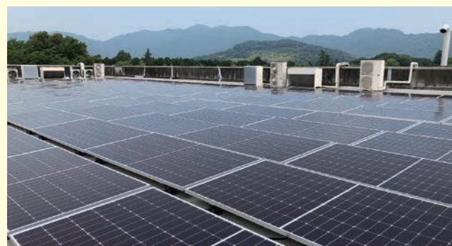
Solar Panel Installation on Roof of R&D Bldg. at Tochigi Plant*3
