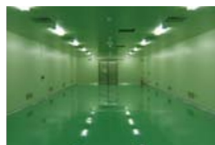
HACCP* clean room facility
