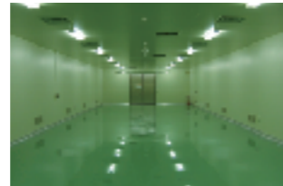
HACCP* clean room facility
