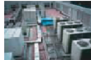
Ice thermal storage facility
