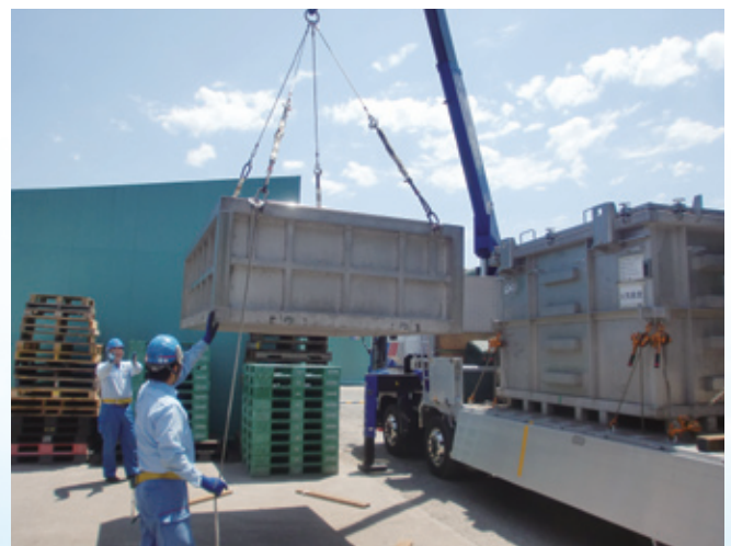
Removal of PCB waste
